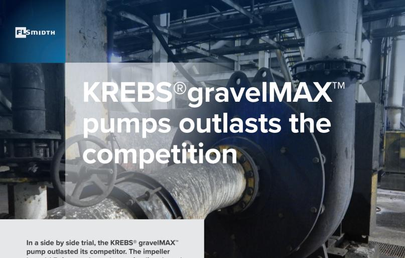
In a side by side trial, the KREBS® gravelMAX™ pump outlasted its competitor. The impeller lasted 1.5 times as long, the suction liner lasted 2 times as long and the casing lasted 2.25 times as long as the competitor's wear parts.
