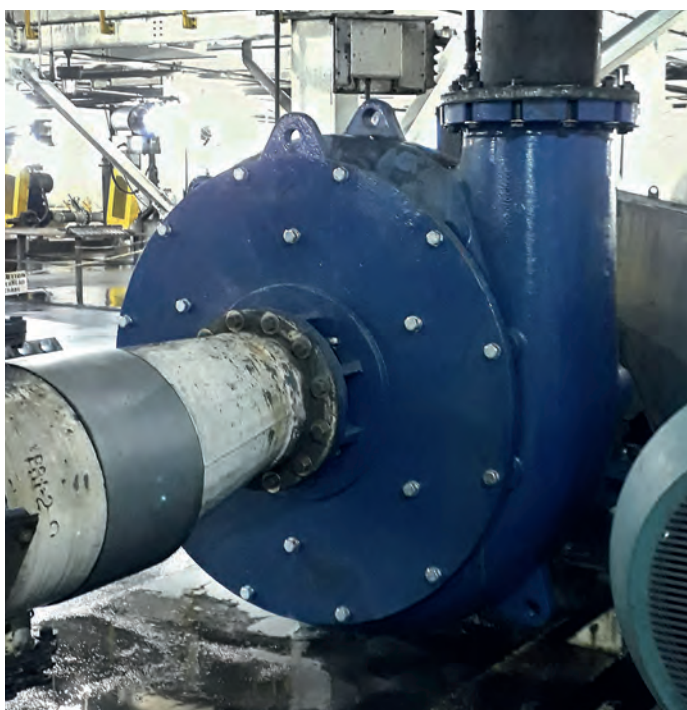
Our gravelMAX pump in a heavy media cyclone feed application in coal processing.
